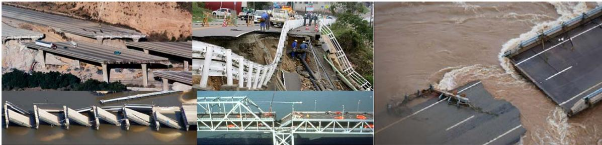
Figure 1: Earthquake-induced (left, middle) and flood-induced damage (right) in road networks.
